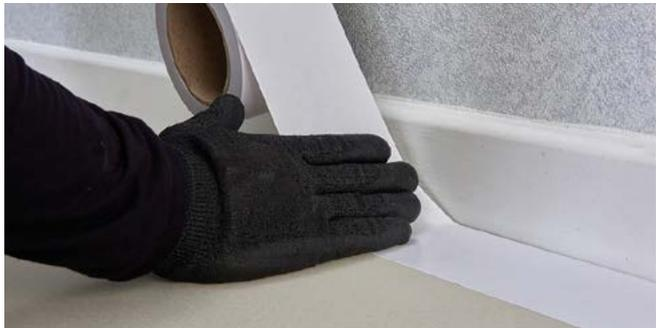
Figure 36 Use double sided QuickLay tape
