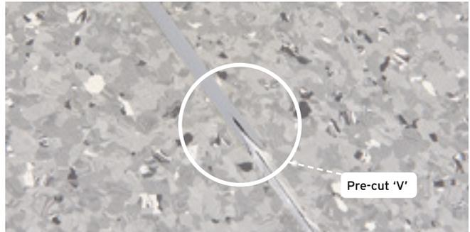
Figure 3 Weld joins
