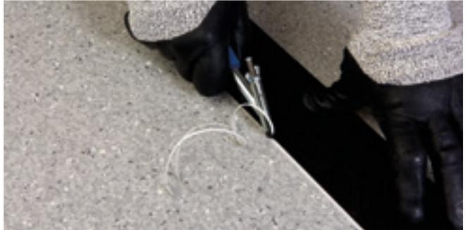
Figure 1 Grooving the seam
