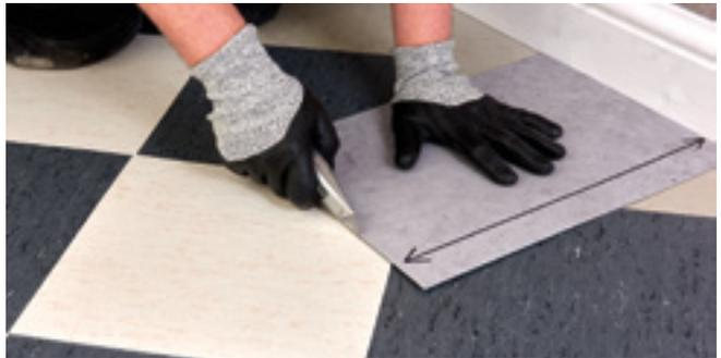
Figure 8 Cutting the perimeter tiles (diagonal cut)
