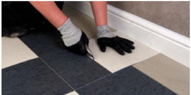
Figure 5 Measuring using an overlapping tile
