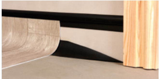
Figure 7 Taper towards a doorway
