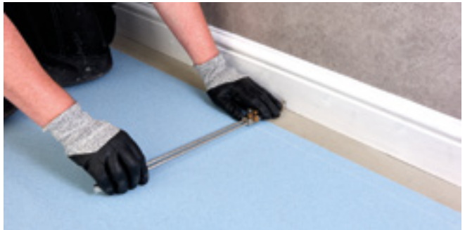
Figure 2 Scribing the wall profile
